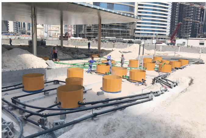
KPS piping's compact electrofusion fittings require the minimum welding time possible
