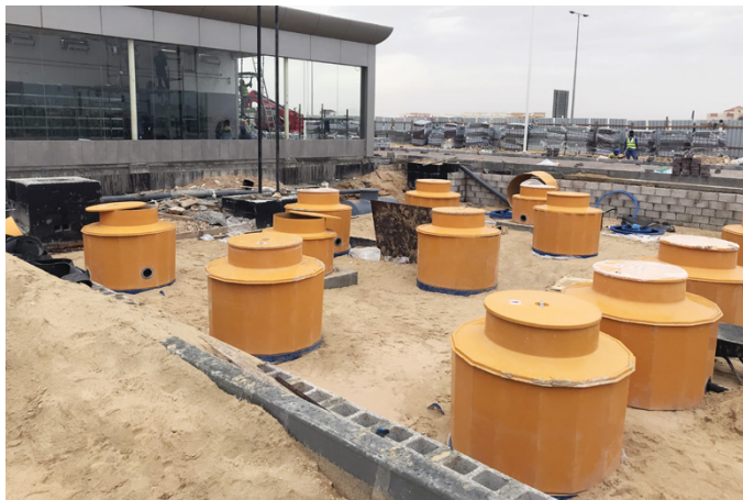
Vacuum testable Fibrelite GRP sumps provide a strong, durable, liquid-tight containment solution
