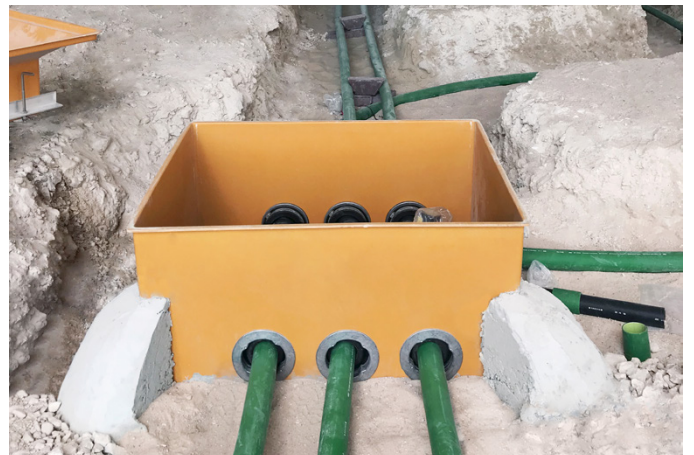
Vacuum testable Fibrelite GRP sumps provided a strong, hard-wearing, liquid-tight containment solution
