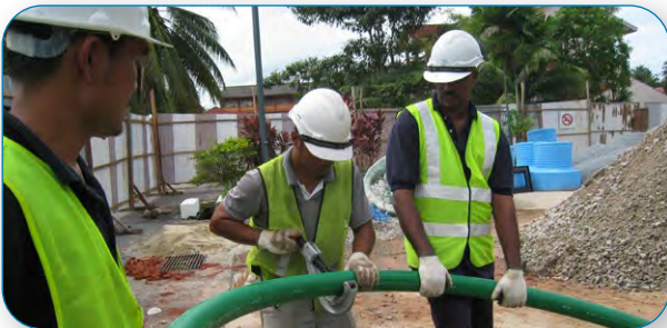
One person should hold the pipe and another do the cutting.
