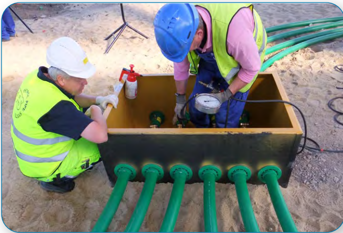
Christian Niejahr OPW Sweden assists an installer on site.
