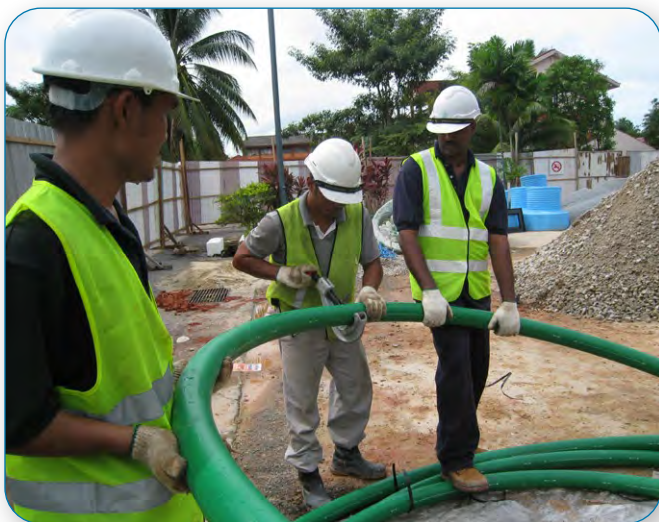
One person should hold the pipe and another do the cutting.
